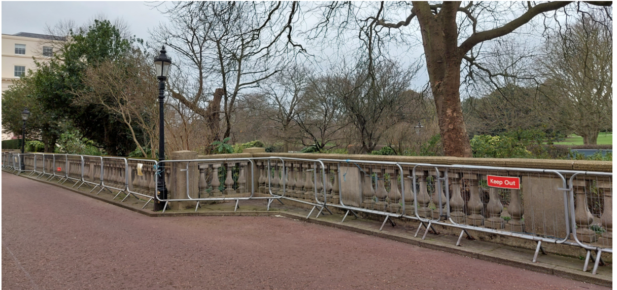
6. Existing wall cordoned off
