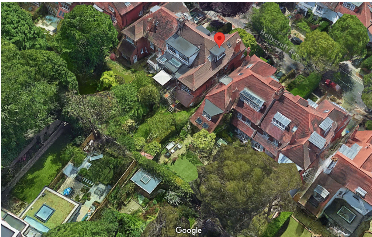
Image 2 (above): Aerial view looking towards rear of property (source: Google)
